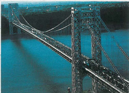
G. WASHINGTON BRIDGE
